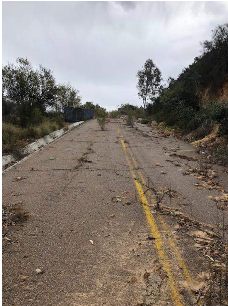
Photo 4. Historic 395 section. Abandoned. Line points in collector as 395-s-002. Facing West. Associated with 1928 route near Pomerado Rd. Road width 21.25 ft. Shoulder overgrown with vegetation.
