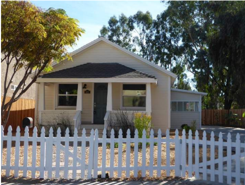
Figure 4.7 443 W. 4th Avenue, looking south at the north façade.
