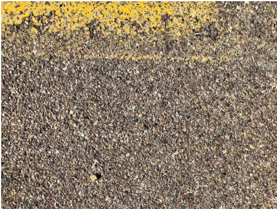
Figure 4.14.5 Close-up of asphaltic paving.
