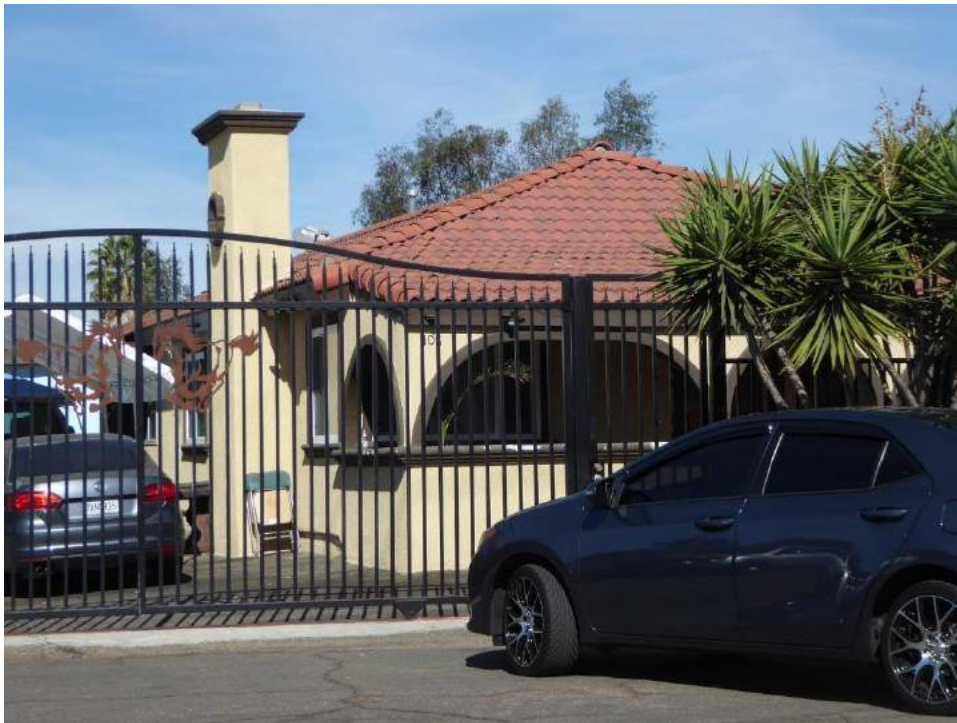
Figure 4.8 408 W. Lincoln Avenue, view of south façade looking northwest.
