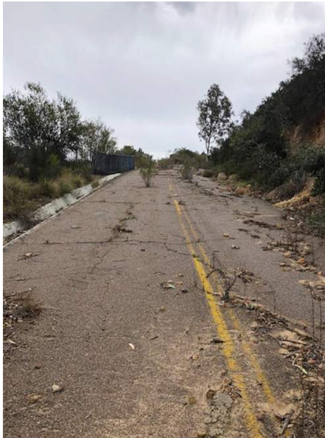
Figure 4.14.3 Abandoned U.S. Highway 395 section, facing west.
