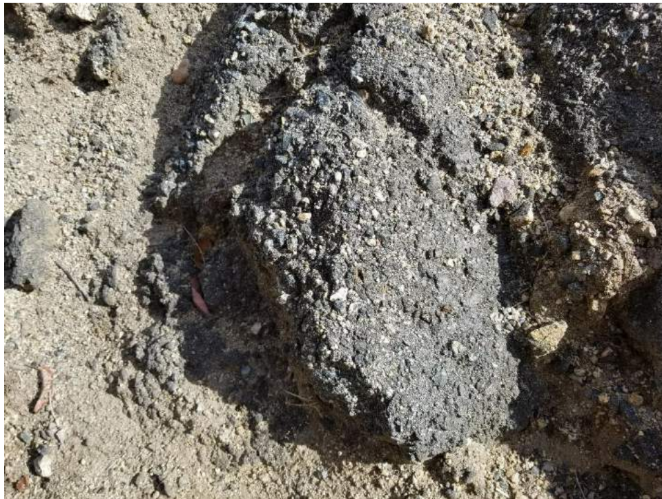
Photo 18. Collector line 395-s-008. Closeup of road material.
