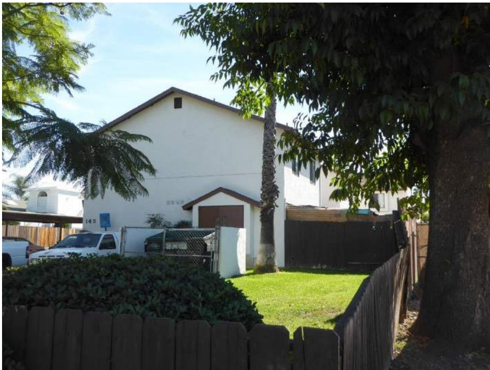
Figure 4.2 South façade of 145 W. Felicita Avenue, looking northwest.
