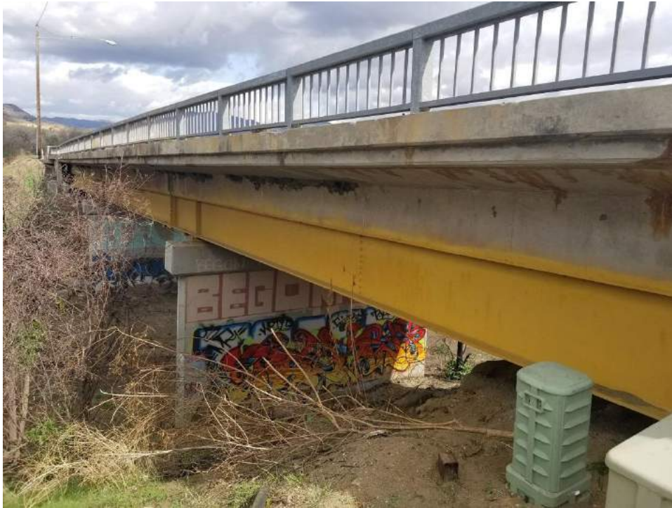
Figure 4.14.22 1947 bridge. Facing northeast.
