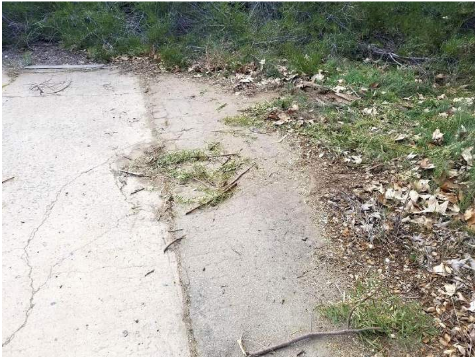
Figure 4.14.15 Photograph shows the concrete roadbed and asphaltic shoulder transition. Facing south.
