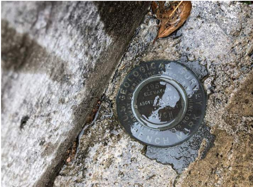
Figure 4.14.7 1955 USGS marker on 1920s-era bridge.
