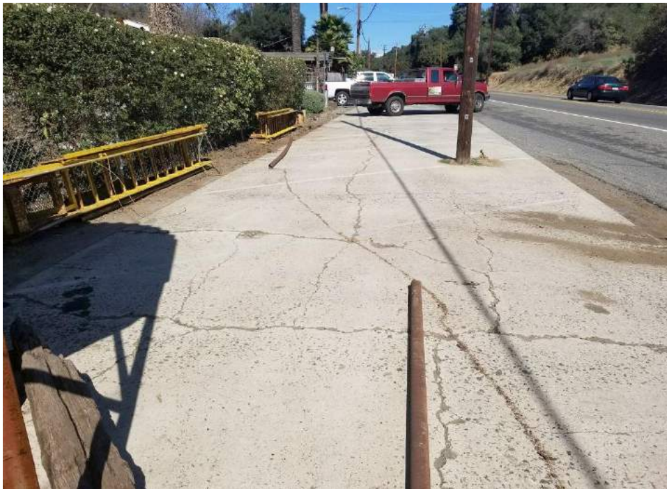
Figure 4.14.9 Abandoned U.S. Highway 395 concrete section, facing north.
