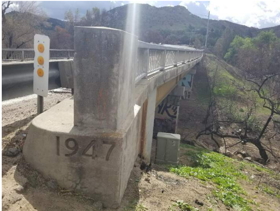
Photo 19. Collector line 395-s-009. 1947 bridge. Facing south. Associated with 1948-1953 section.
