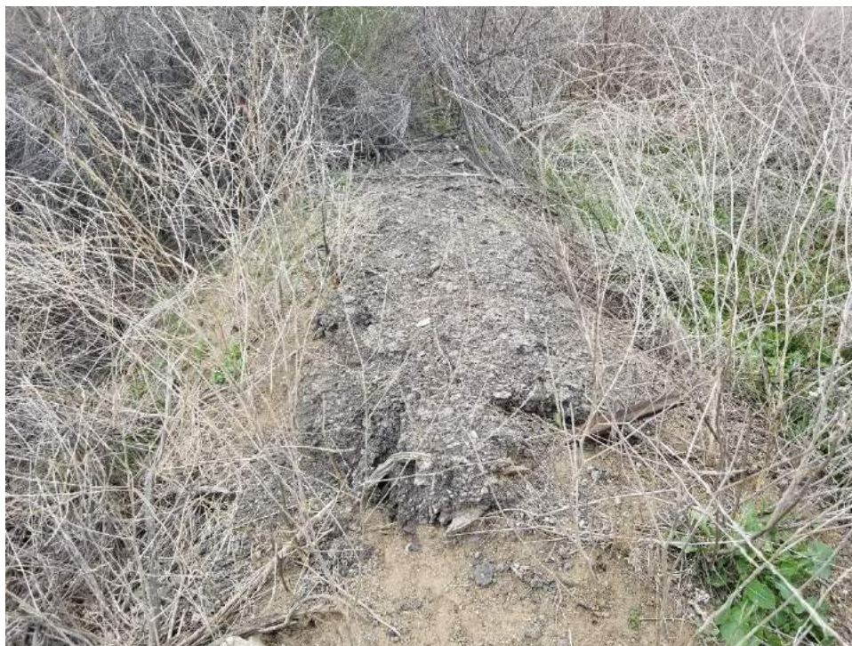
Photo 16. Collector line 395-s-007. Closeup of asphalt material.
