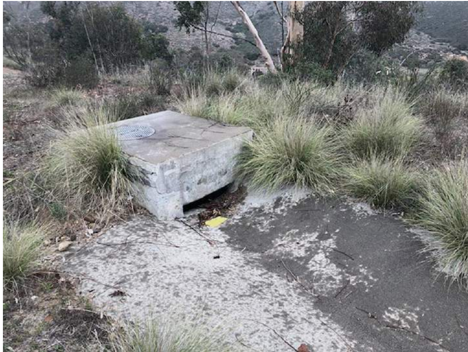
Figure 4.14.1 Possible historic drain clean out associated with the 1935-1947 route. Facing southeast.
