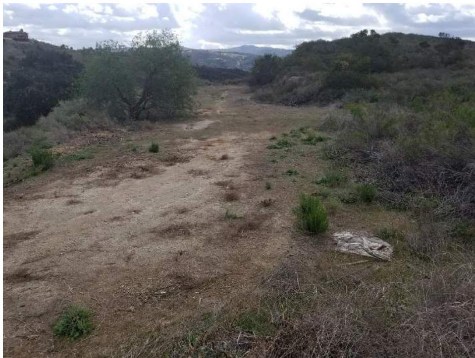
Photo 14. Collector line 395-s-007. Mostly cleared except for a very small area of asphalt that appears in situ, and broken asphalt rubble elsewhere. Facing southeast. Associated with 1948-1953 section.
