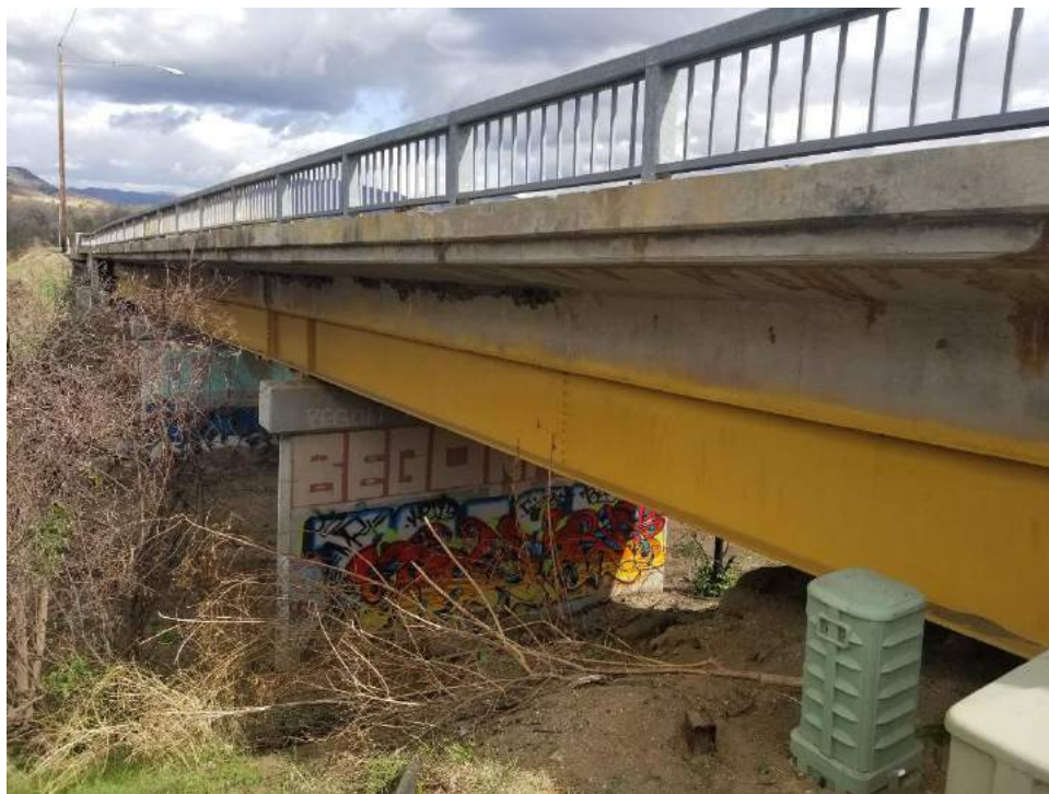
Photo 20. Collector line 395-s-009. 1947 bridge, facing northeast. Associated with 1948-1953 section.
