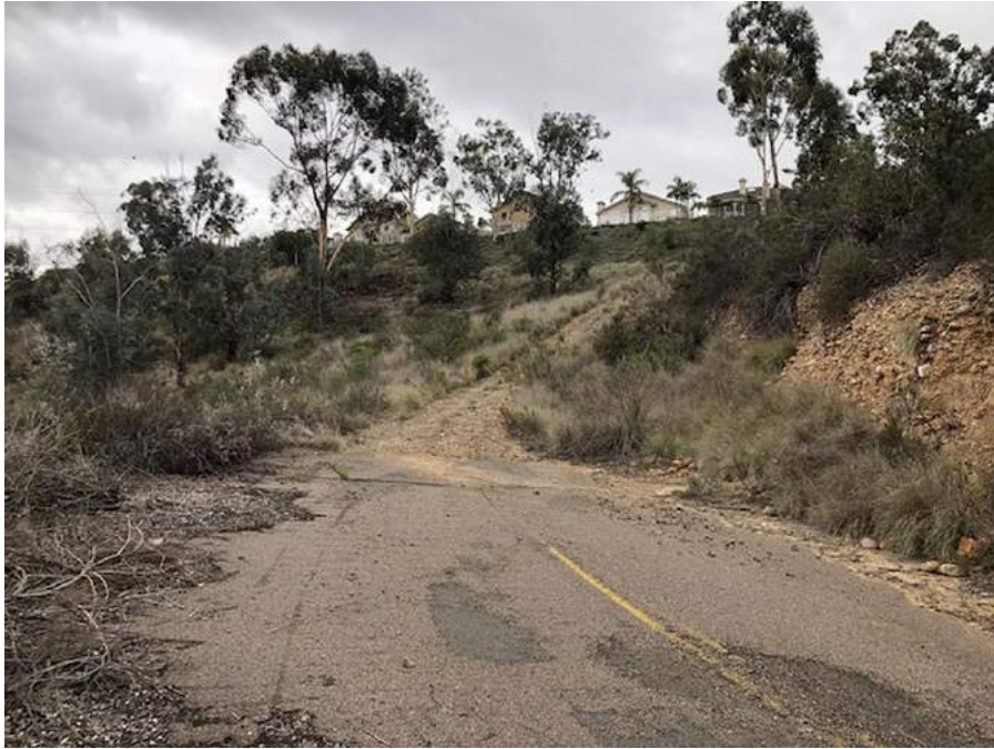
Figure 4.14.2 Abandoned U.S. Highway 395 section, facing northwest.
