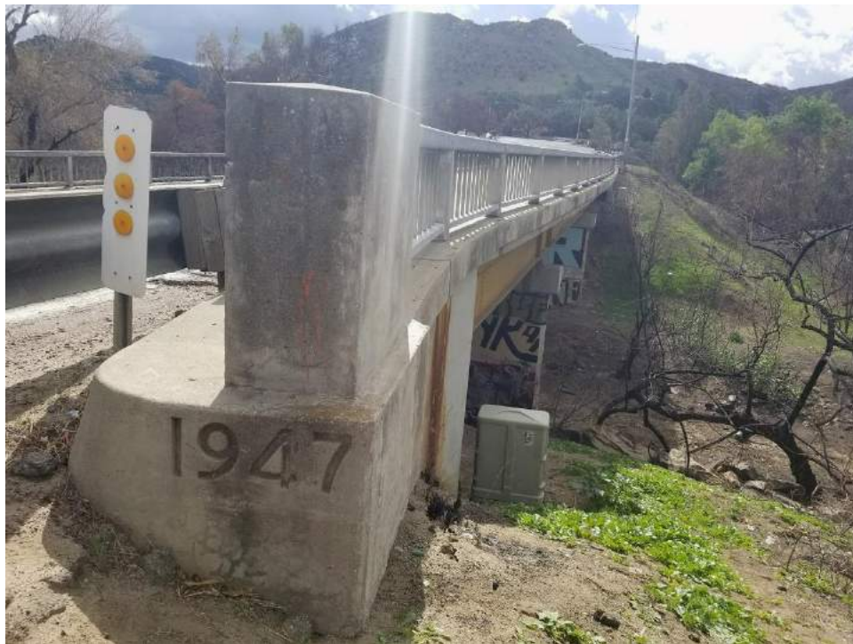
Figure 4.14.21 1947 bridge. Facing south.
