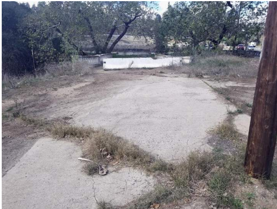
Figure 4.14.11 Concrete road segment and bridge. Facing northwest.
