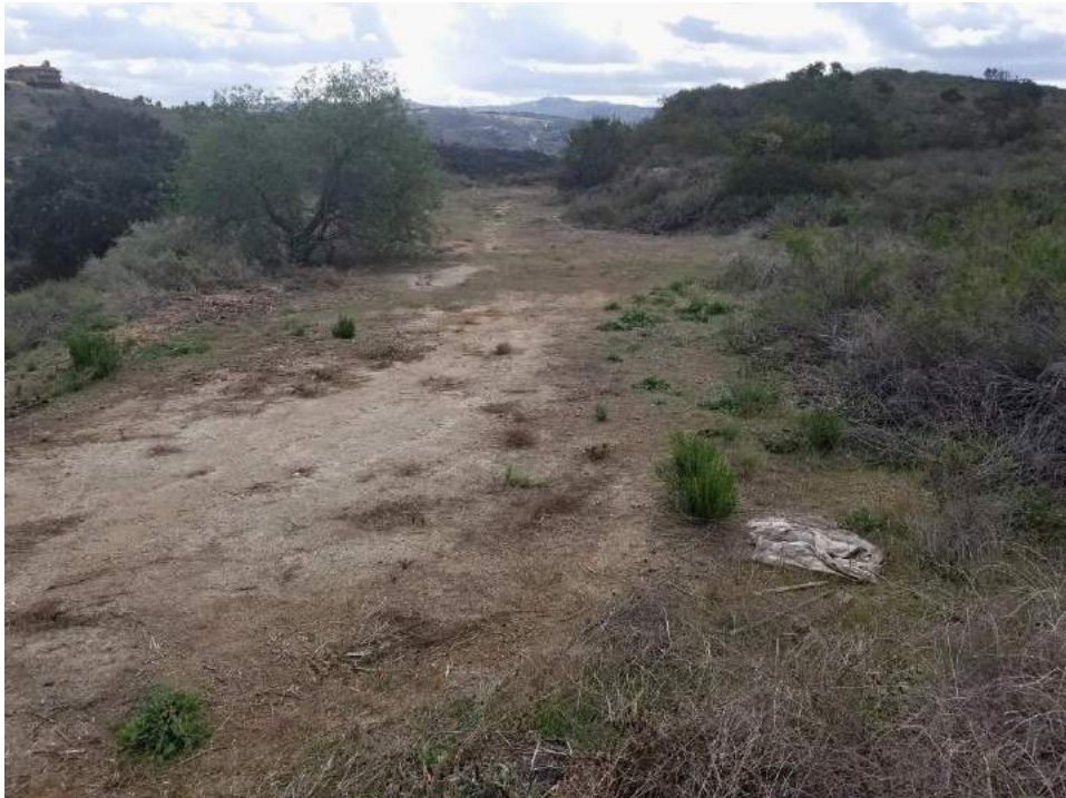
Figure 4.14.16 This abandoned segment was mostly cleared except for a very small area of asphalt that appears in the ground with broken asphaltic rubble elsewhere. Facing southeast.
