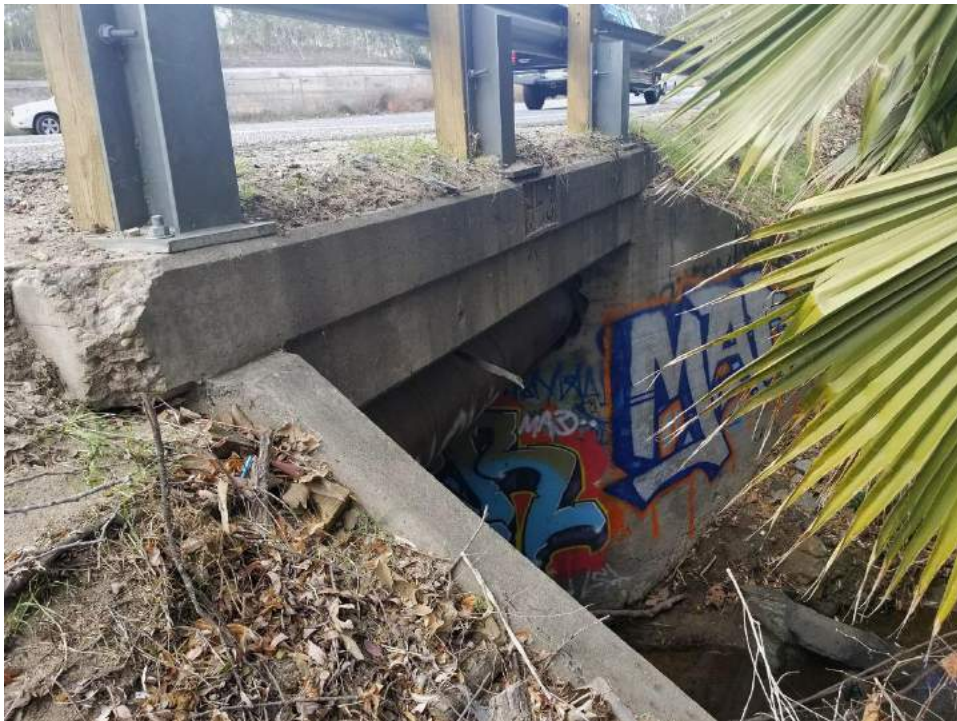
Figure 4.14.13 1943 culvert. Facing northwest.
