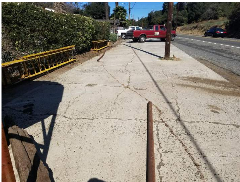
Photo 12. Collector point 395-s-005. Historic road section remnant, 18 feet wide, used as business parking. Photo facing North. Associated with 1928 route.
