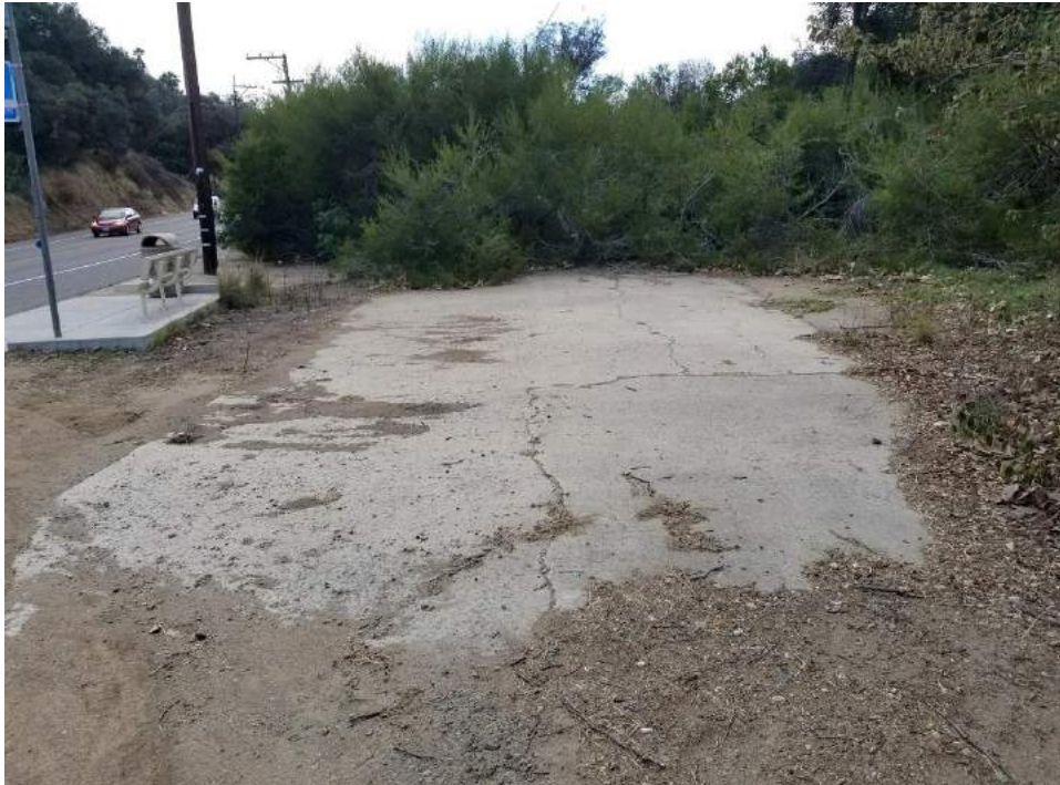
Figure 4.14.14 This concrete segment is 28 ft. 9 in. wide. Asphaltic shoulders vary with 5 ft. 10 in. as the widest. Facing south.
