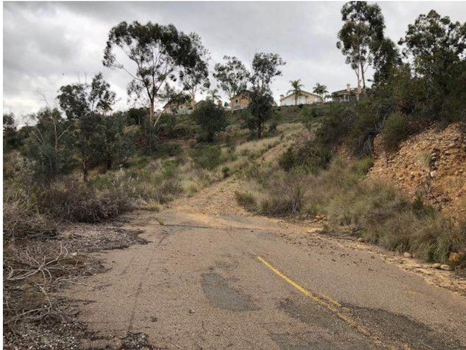
Photo 3. Historic 395 section. Abandoned. Line points in collector as 395-s-002. Facing NW. Associated with 1928 route near Pomerado Rd. Road width 21.25 ft. Shoulder overgrown with vegetation.
