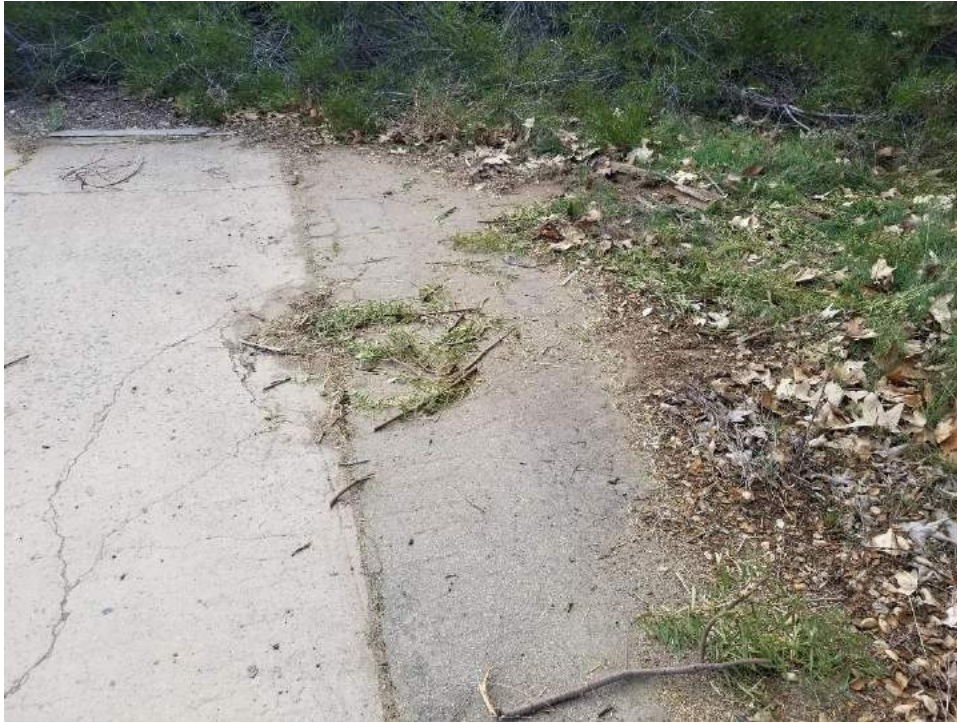
Photo 25. Collector line 395-s-012. Closeup of concrete and asphalt.
