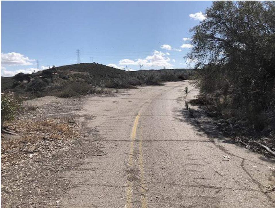
Figure 4.14.4 Abandoned U.S. Highway 395 section, facing west-southwest.
