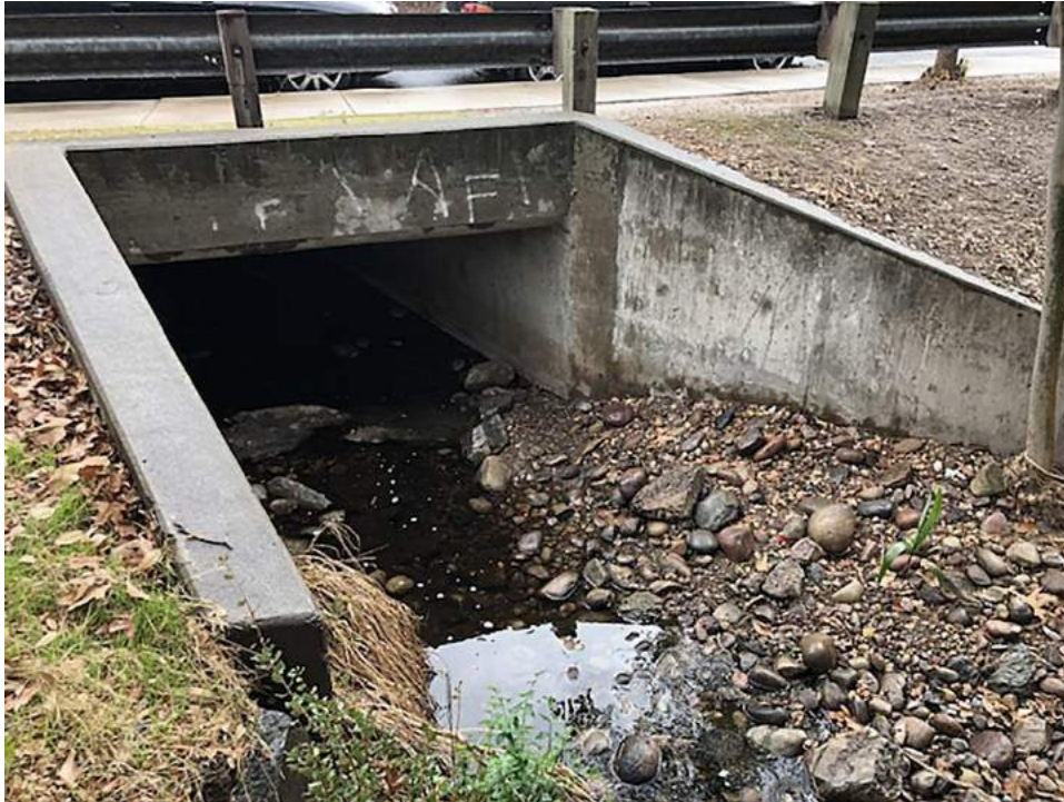
Figure 4.14.8 Possible historic culvert. Facing southeast.
