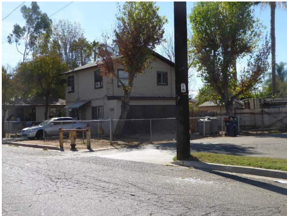
Figure 4.6 View looking southwest at the east façade of 733 S. Pine Street.
